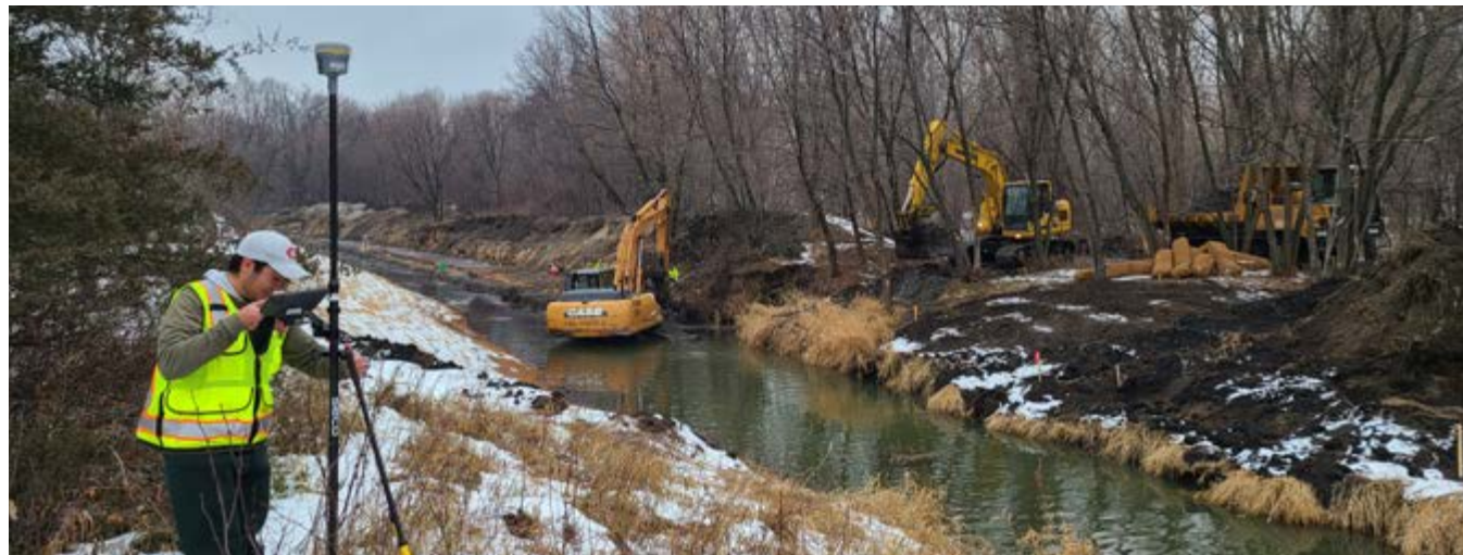
Field Operations Manager completing a survey at the Coon Creek Park Stream Restoration Project site
