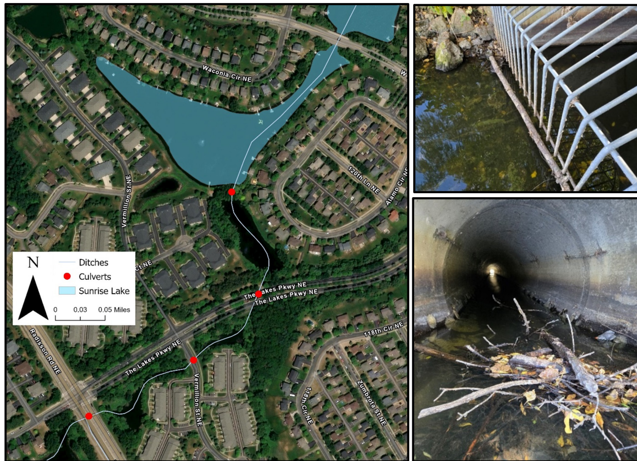
Figure 7. Locations of Sunrise Lake outlet and downstream culverts (left). Image of Sunrise Lake outlet structure showing trash rack and culvert (upper and lower right).
