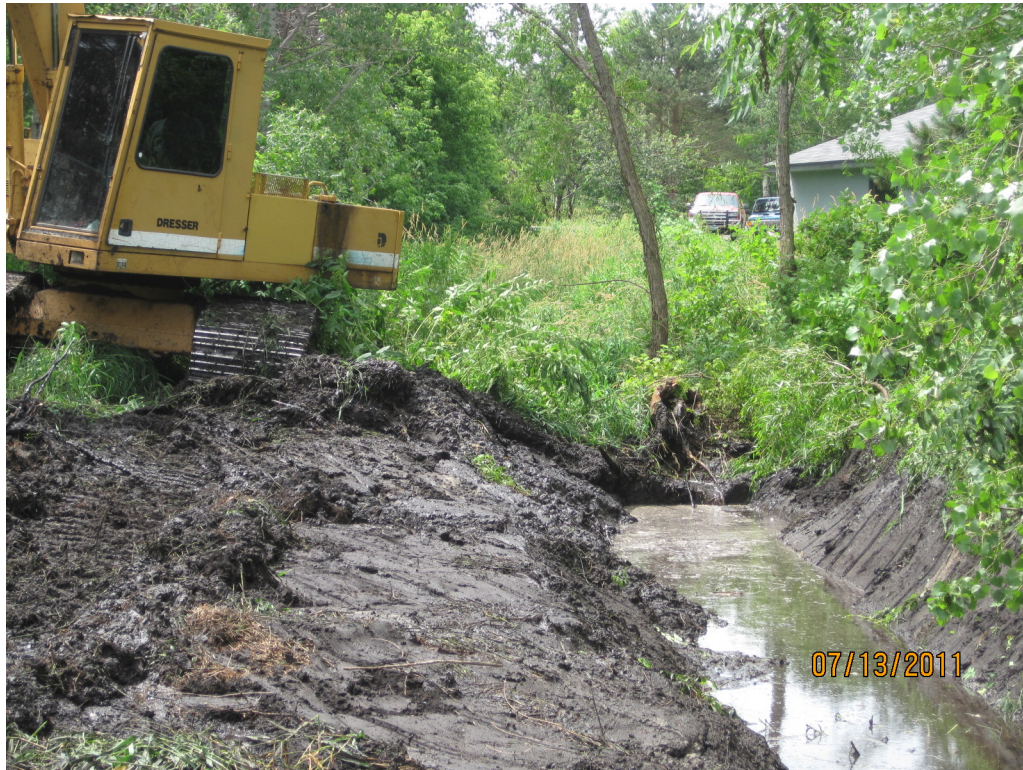
Ditch 58-7-3 at Constance Cleaning 2011
