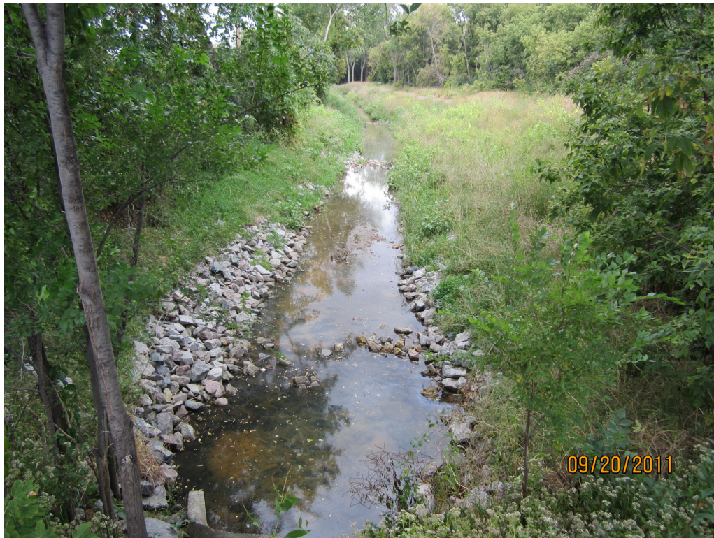
Woodcrest Creek Rehabilitation Inspection off Foley (Installed 2010)
