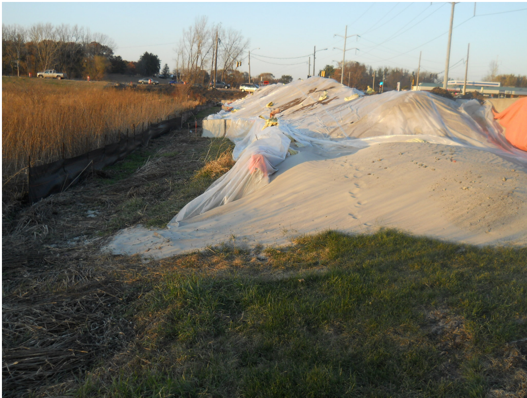
Perimeter control needed for Hwy 242 reconstruction in Blaine
