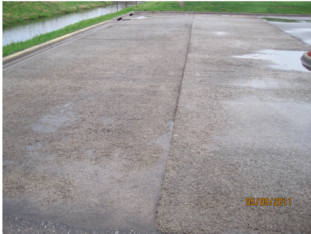
National Sports Center Pervious Pavement Inspection (Installed 2010)
