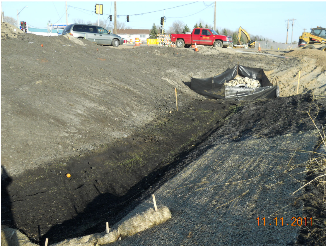
Inspection southwest of Jefferson Street and 242 reconstruction
