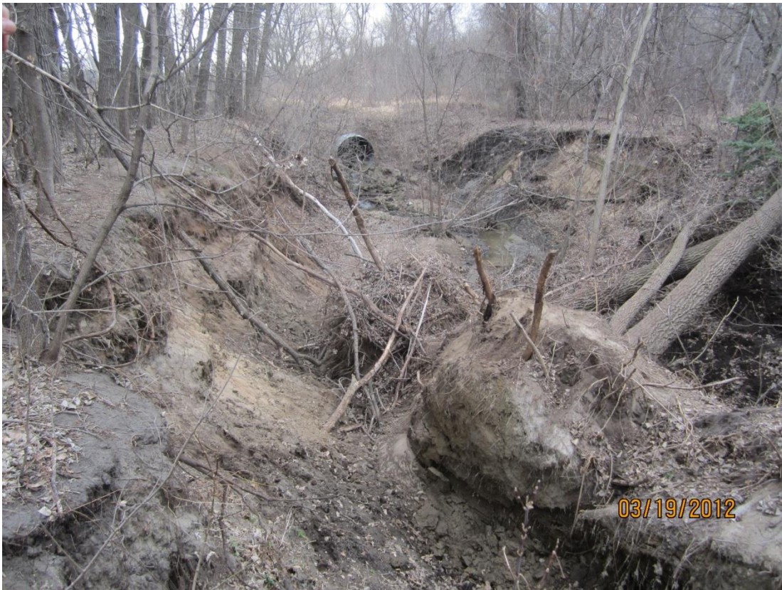
Woodcrest Bank Erosion and fallen Cottonwood Tree
