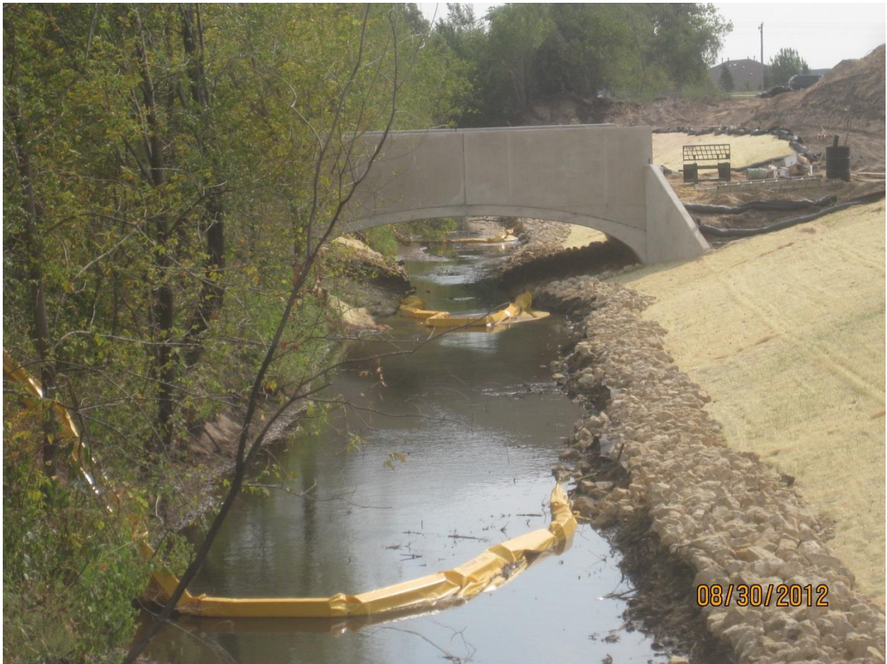
Stabilization of ditch banks and channel protection, Wal-Mart of Blaine
