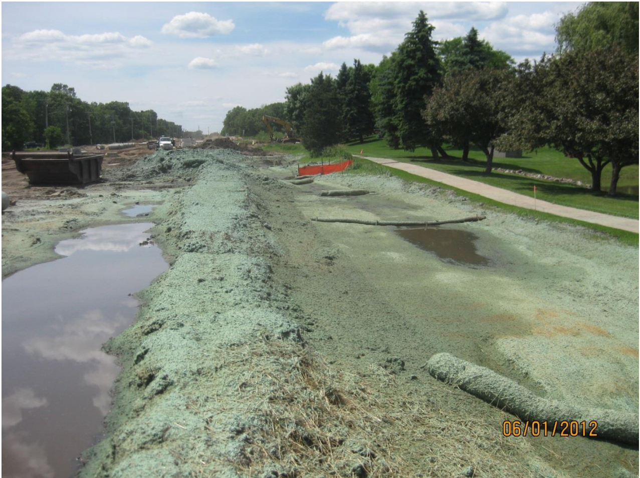
Inspection southwest of Jefferson Street and 242 reconstruction, Coon Rapids
