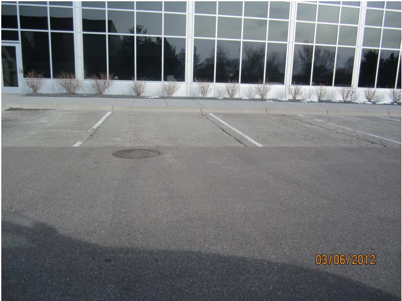
City of Blaine Public Works Facility Pervious Pavement Inspection (Installed 2010)
