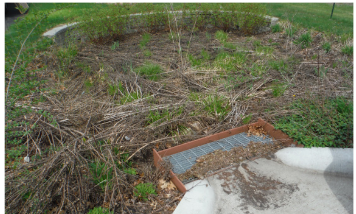
The matted brown vegetation in this rain garden needs to be removed. The Rain Guardian pre-treatment device needs to be cleared of debris. The inner chamber should be cleaned out: remove its top grate to shovel out the inner chamber and then remove the inner filter and clean it.
