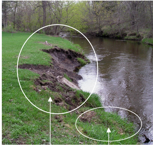
Mowing to edge. Bank is slumping.
