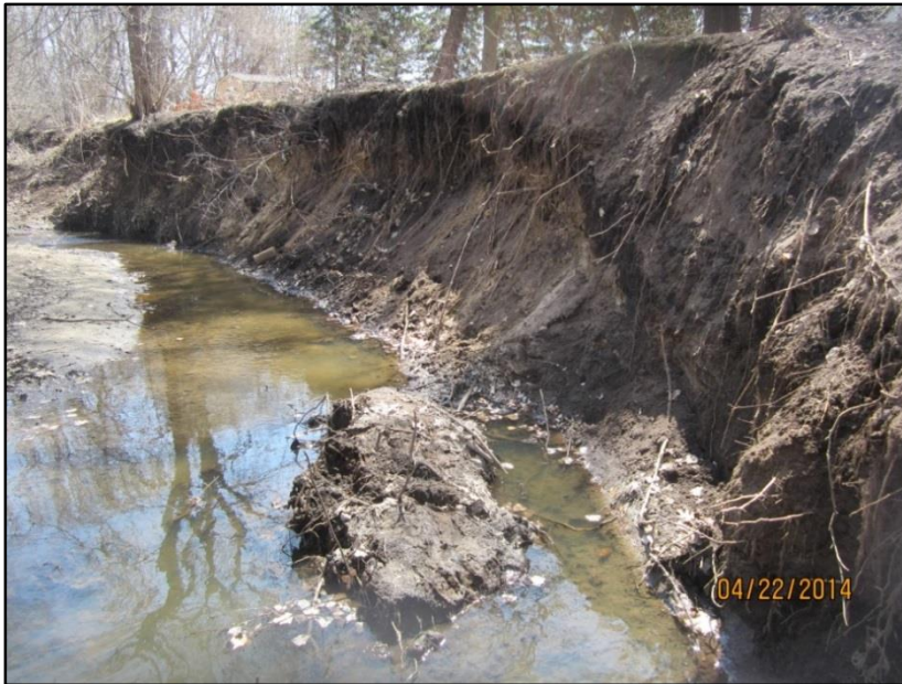
Figure 11. Streambank erosion in Coon Creek Subwatershed.
