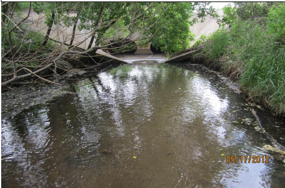
Fish barrier on upstream end of Evergreen Blvd.
