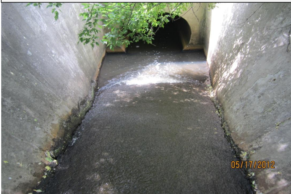
Fish barrier on upstream end of Holly Street NW.
