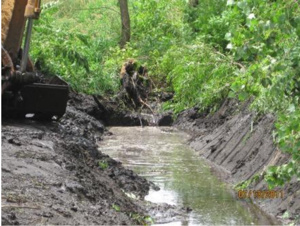
Figure 37. Channel in the process of being dredged.
