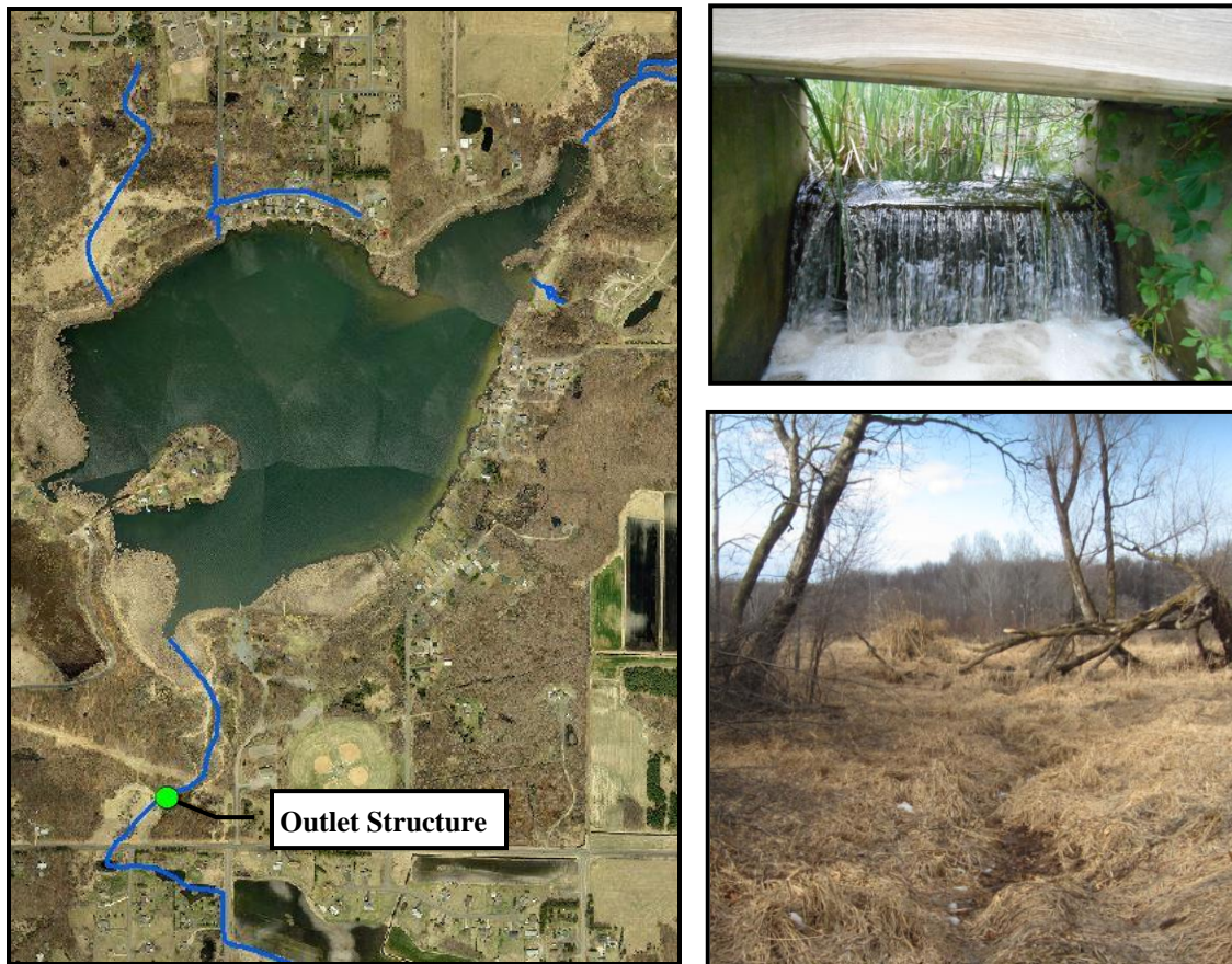
Figure 4. Location of the Ham Lake outlet and photographs of the box culvert during wet conditions (upper right) and the channel looking upstream of the outlet structure during dry conditions (lower right).
