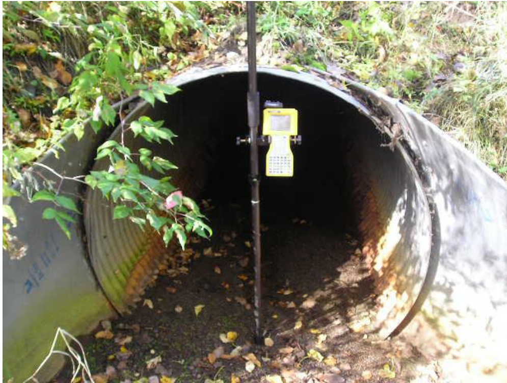
Culvert inspection Ditch 58
