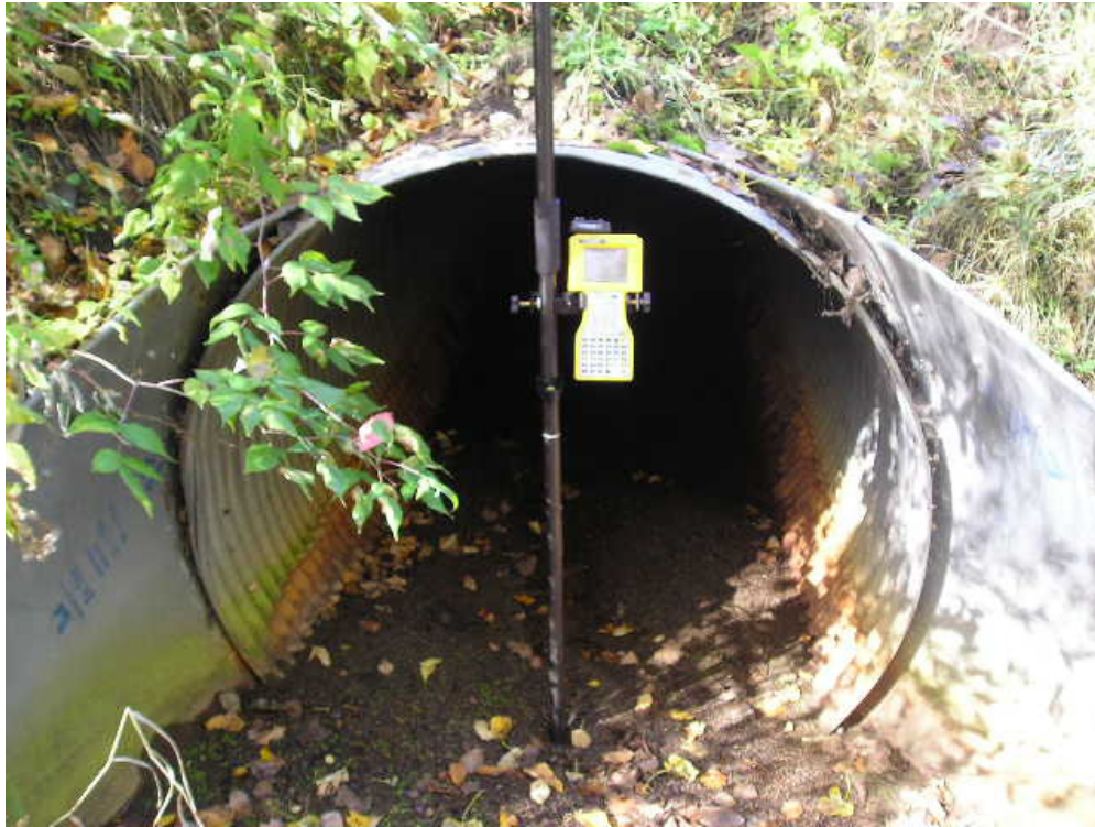
Culvert inspection Ditch 58
