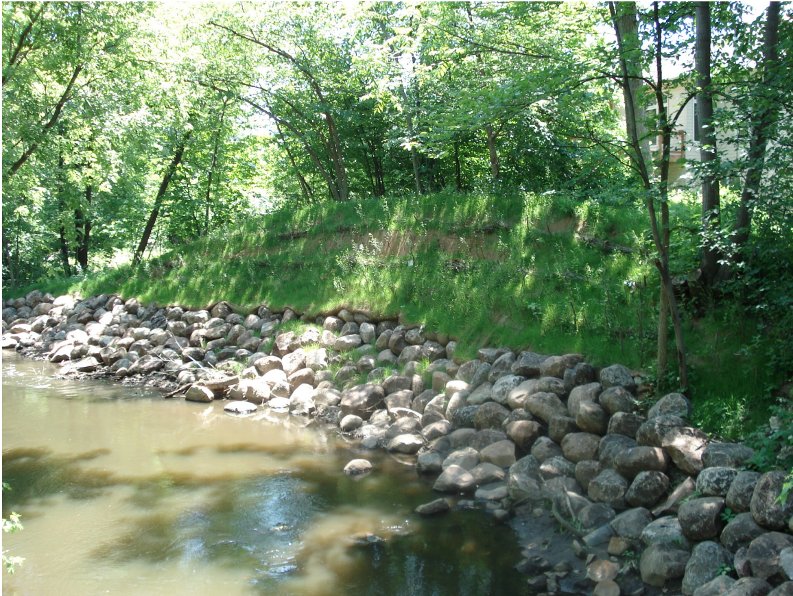
Kar bank stabilization spring 2008
