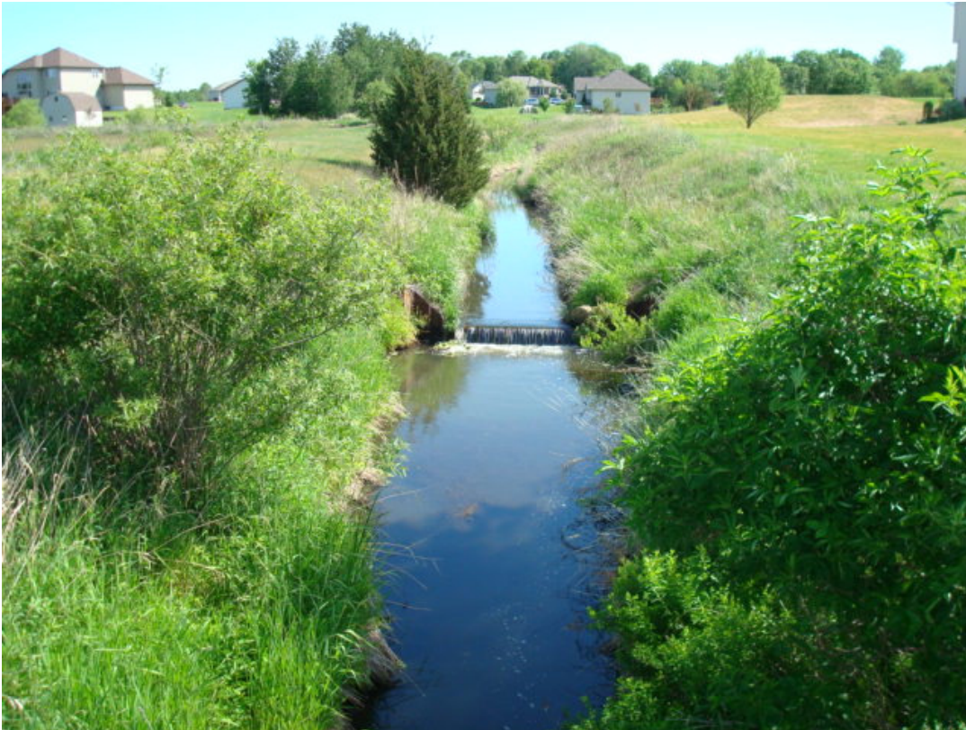
Structure on Ditch 58
