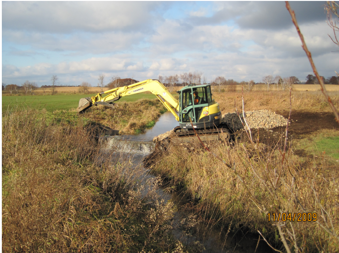
Timberline Structure Repair, 2009
