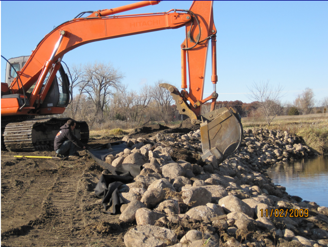
Crown Point bank stabilization fall 2009
