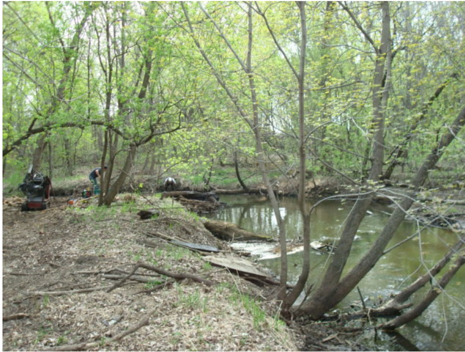
Clearing downed trees at Erlandson Park, May 2009
