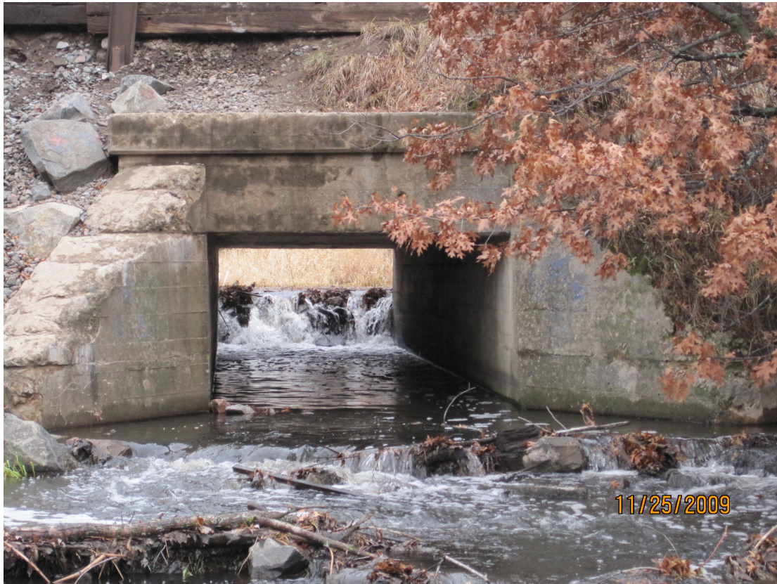
Dam on Sand Creek (Ditch 41), Coon Rapids, November 2009
