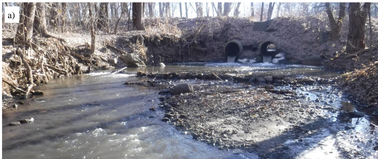
Figure 2. Photos of aquatic organism passage concerns and active erosion at two of the candidate sites: a) undersized, perched culverts at Sand Creek at Xeon Boulevard crossing with scour and bank sloughing, b) active bank erosion immediately downstream of Sand Creek at Xeon Blvd crossing, c) undersized culverts at Lower Coon Creek Service Road crossing that create a velocity barrier during high flows and are prone to clogging, d) active bank erosion immediately upstream of Lower Coon Creek Service Road crossing.
