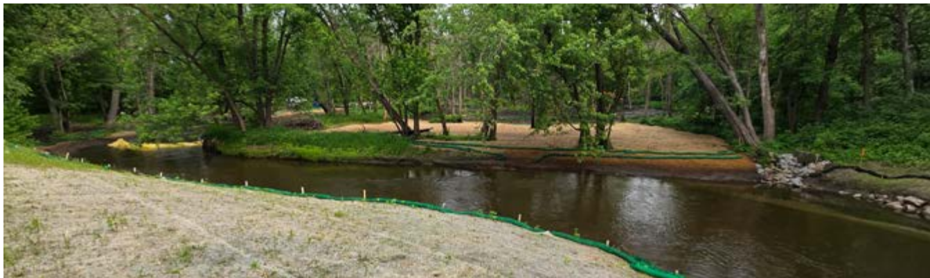
Portion of Lower Coon Creek Corridor Restoration Project site during stabilization
