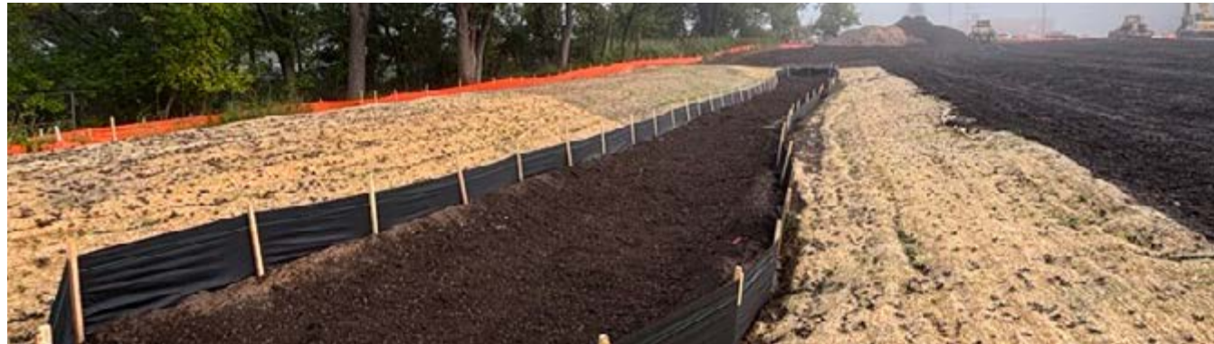
Construction site erosion control practices around an infiltration basin (black fencing) and site perimeter (orange fencing)
