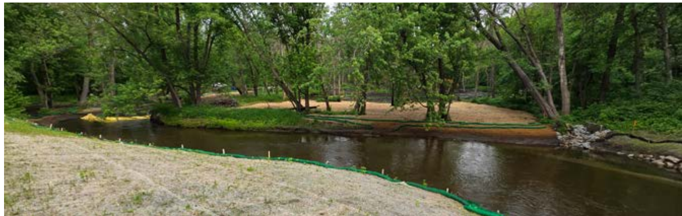
Portion of Lower Coon Creek Corridor Restoration Project site during stabilization
