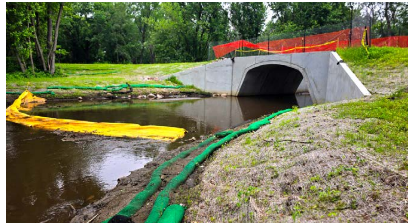
Freshly installed pedestrian bridge with open bottom culvert
