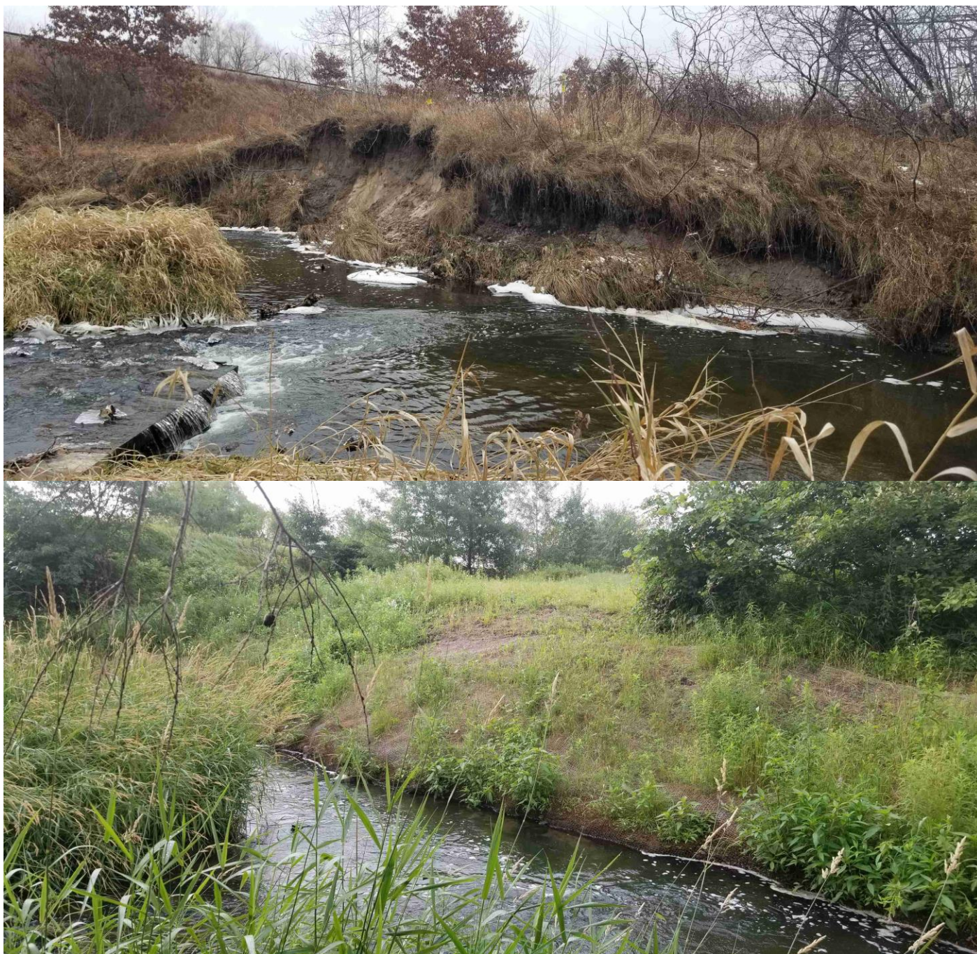
An eroded bank before and after stabilization with vegetated riprap
