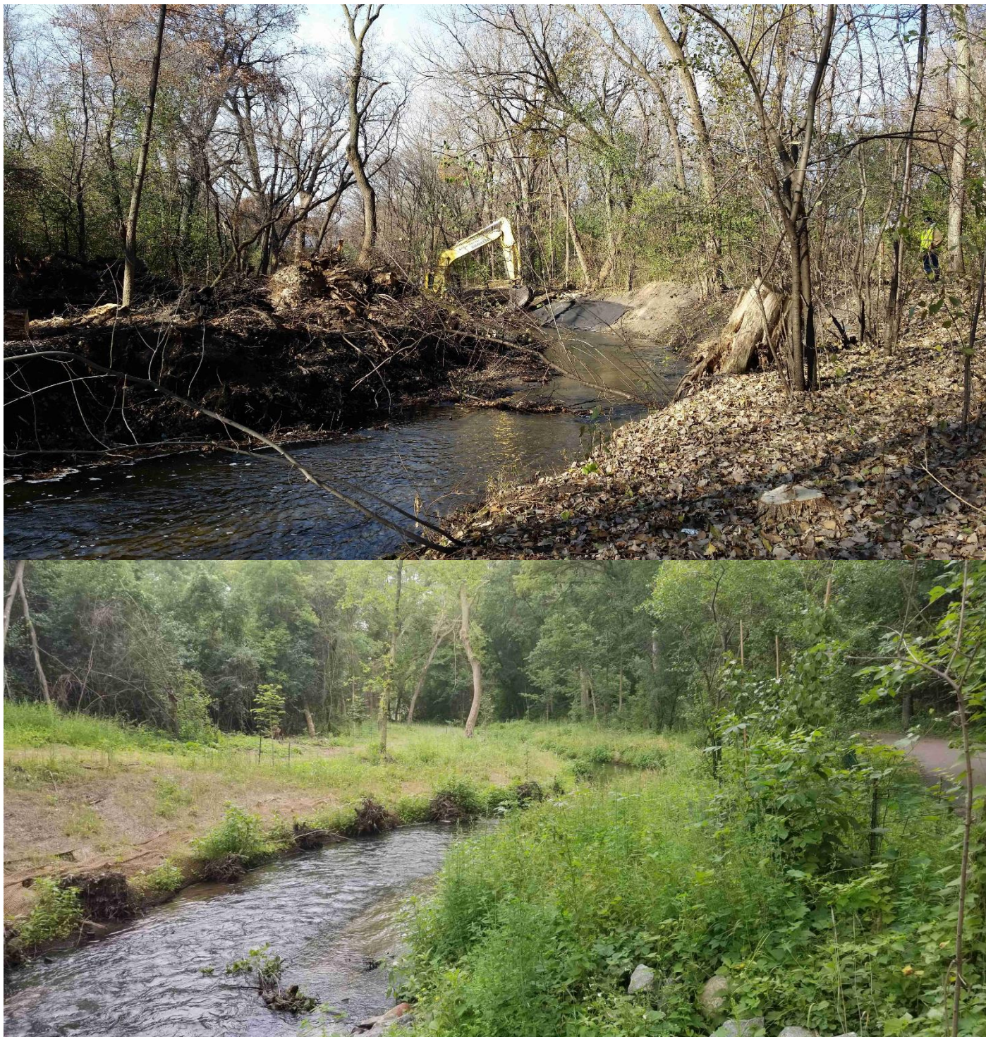
An eroded bank before and after stabilization with log toe and root wads
