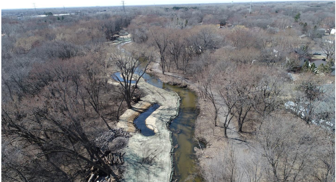
Drone imagery of the project reach after the first phase of construction. Several newly constructed partial meanders are shown on the left with Sand Creek continuing to flow in its former alignment on the right. The site was left inactive for the 2020 growing season to promote revegetation/stabilization of the constructed meanders before excavating the rest of the new channel and diverting flow into it during winter 2020-2021.
