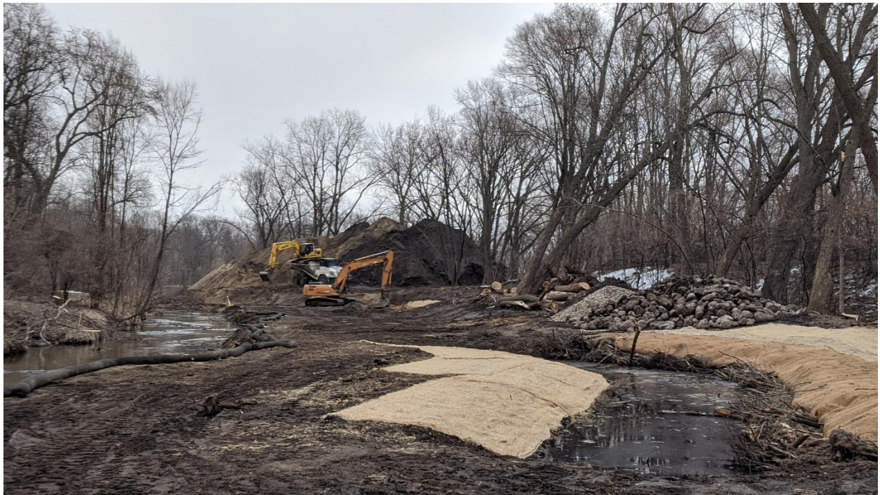
Construction of a new meander stabilized with toe wood shown on the right during the first phase of construction in Winter 2019-20. Partial meanders were constructed off-line with stream flow still routed down the former channel (left).
