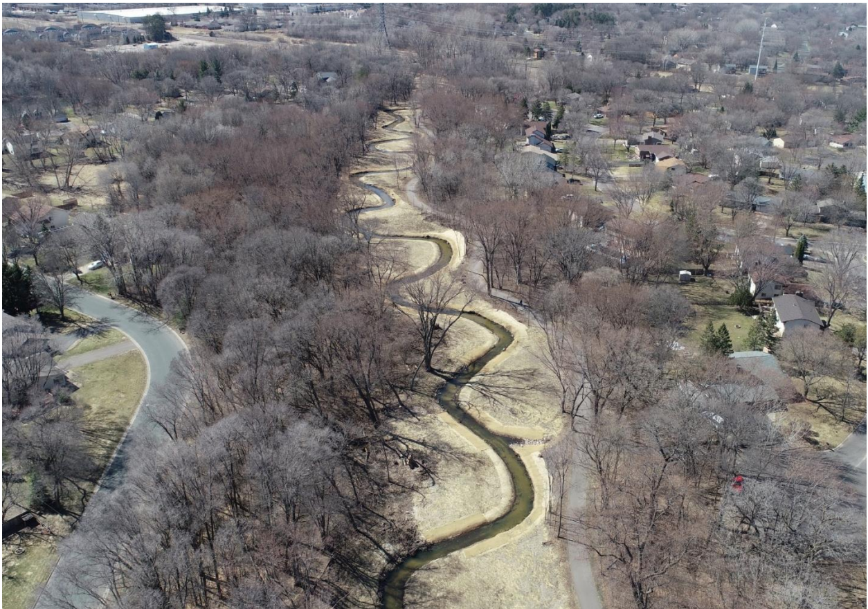
Drone imagery of the newly constructed meandered channel in Spring 2021.
