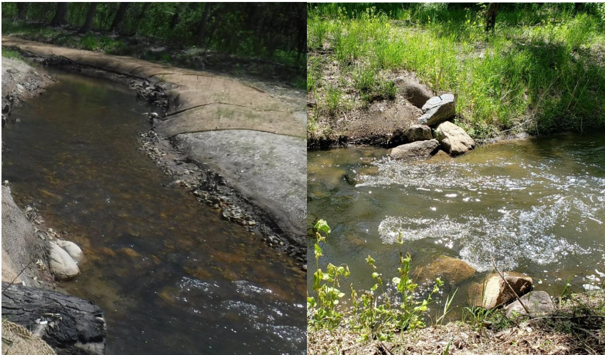
An engineered gravel riffle paired with a boulder cross vane to halt stream bed incision and create riffle-pool sequencing for improved in-channel habitat. Six gravel riffles and nine cross vanes were installed within the project reach.
