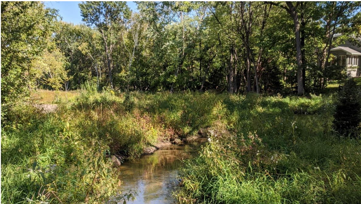
View of newly constructed channel from the same vantage point in April 2021 (upper) versus August 2021 (lower) showing revegetation progress. Despite drought conditions in 2021, native seed and planted live stakes and trees flourished, enhancing riparian habitat and helping to stabilize banks.
